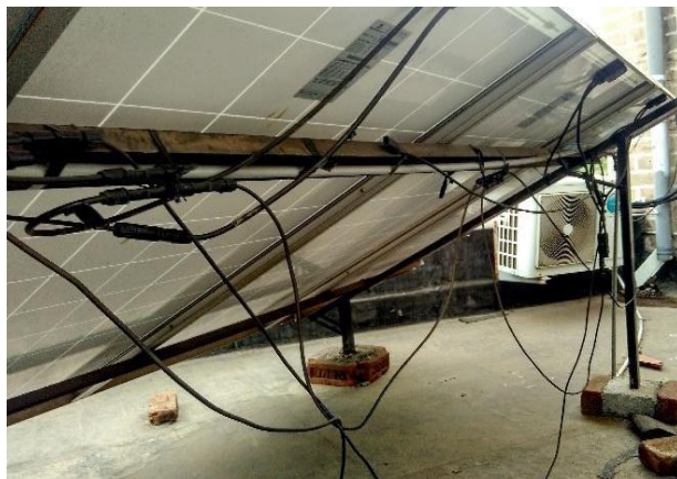
Figure 4: Four panels connected in parallel
