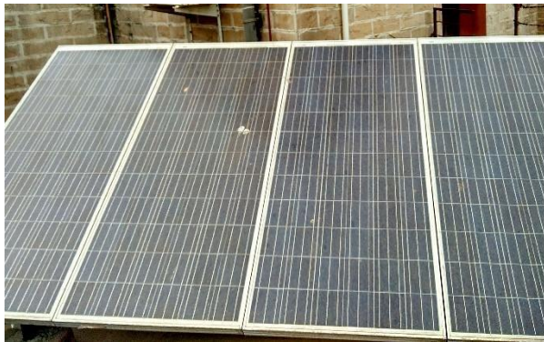
Figure 3: Front view of TP-280 PV panels
