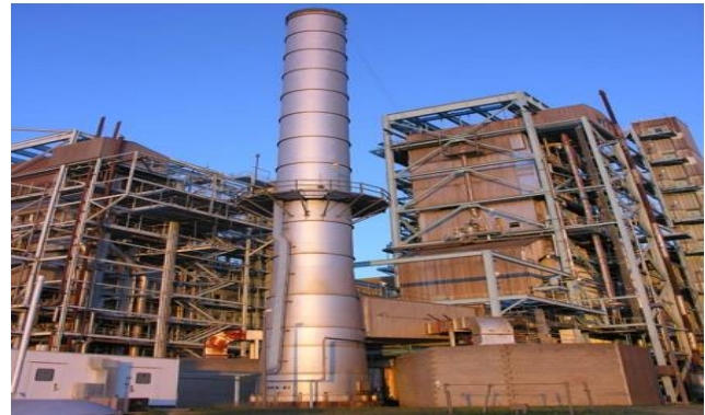
Figure 1.1 cantilever steel chimney
